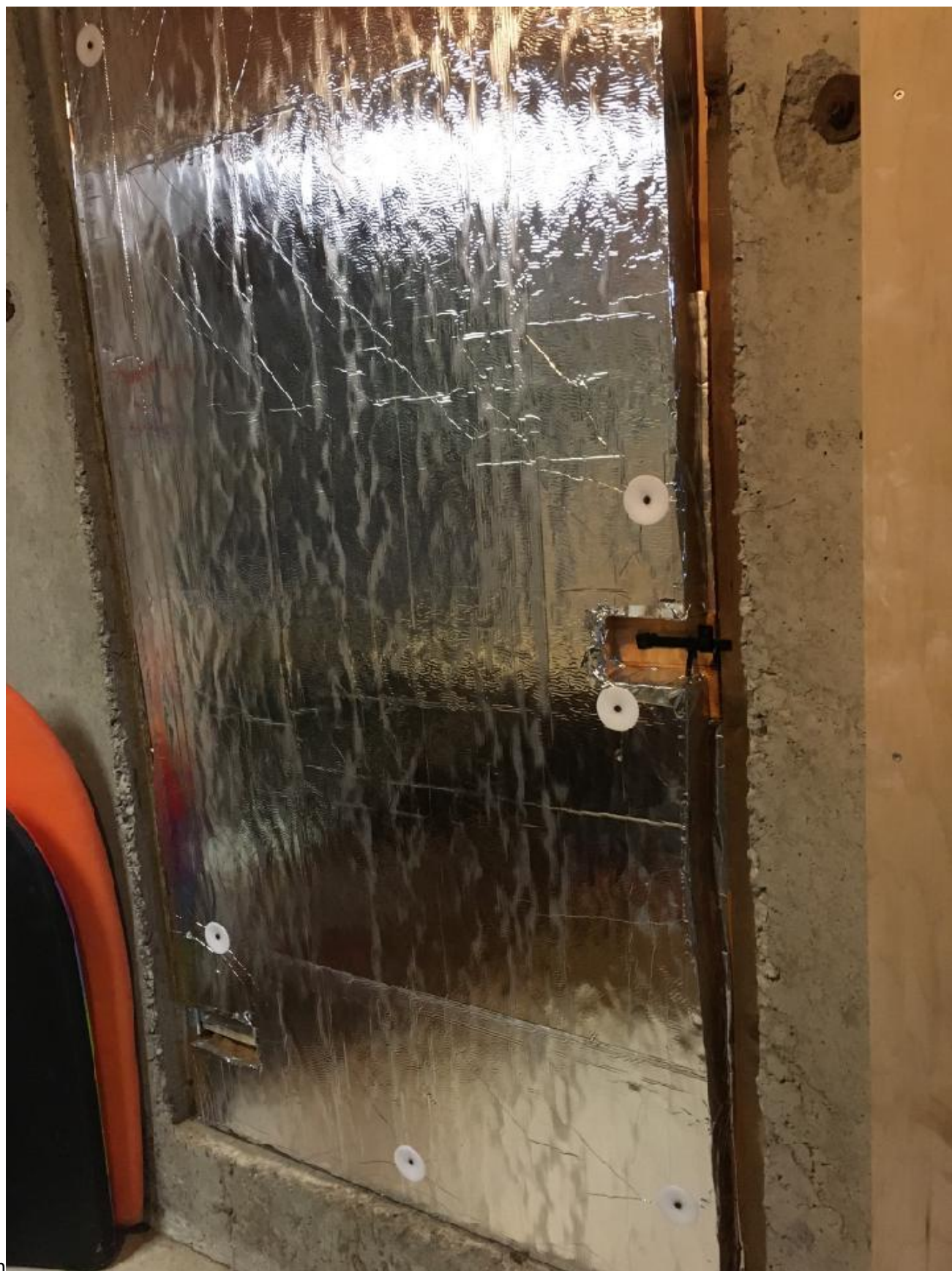
In Insulation on basement door
