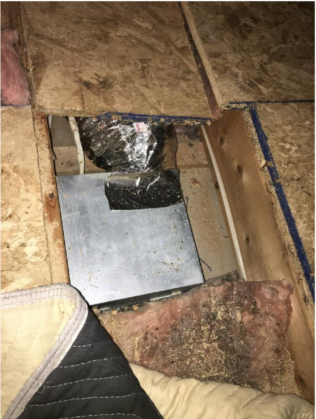
2 Bathroom vents were insulated
