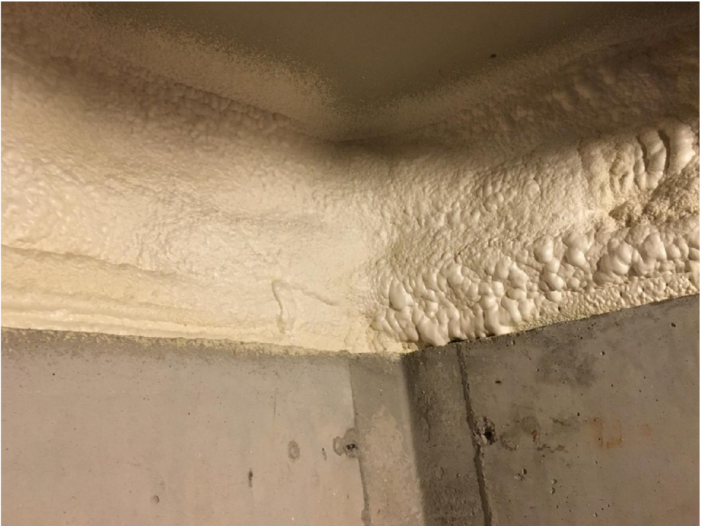
Basement junction with wall above. This was also done around the floor junction with basement walls.
